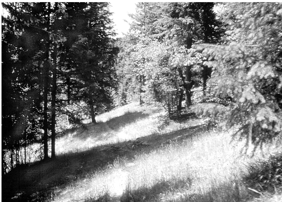
Road recontouring (middle of photo) along Grass Valley Creek in Redwood National Park, northern California, one year after project completion. The removal of roads and recontouring of slopes helps restore hydrological processes and aquatic health while reducing the effects of forest fragmentation. Photo by John McCullah, Salix Applied Earthcare
