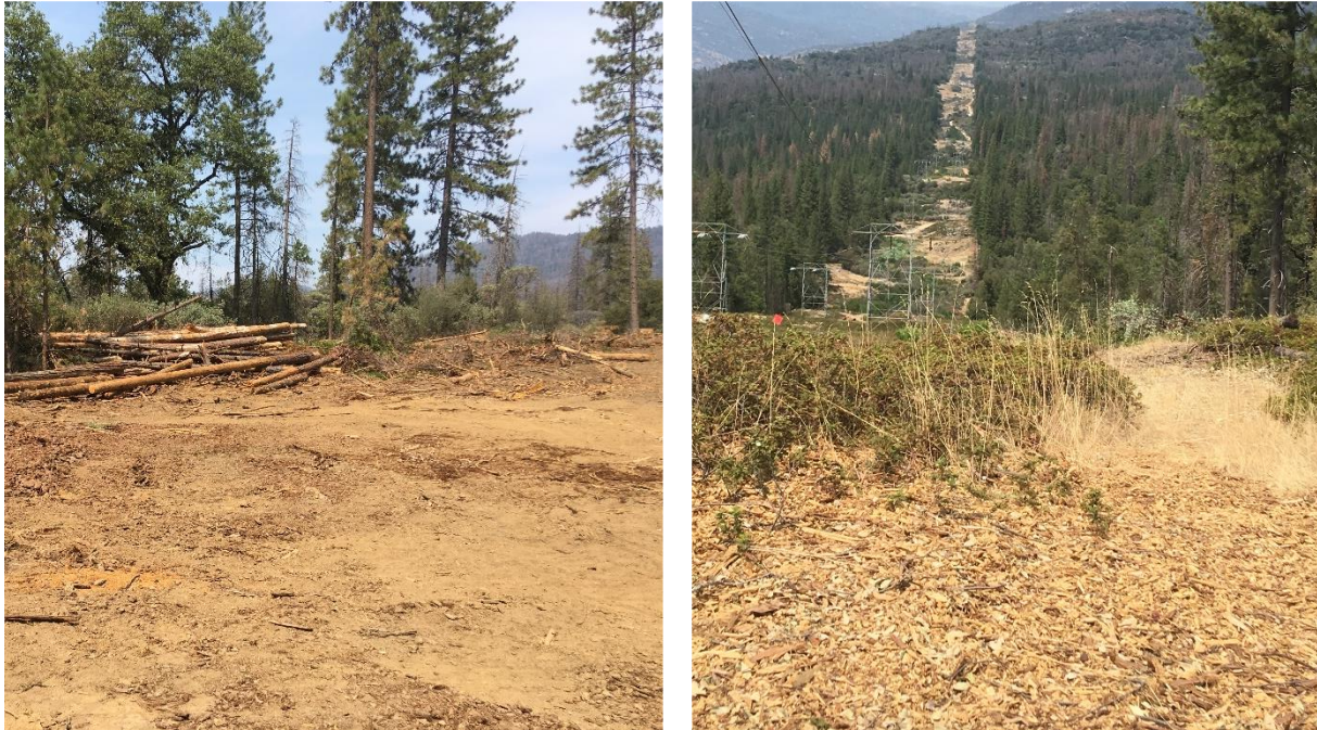
Figure 3: Musick Area: Road 9s07b & Existing Fuelbreak under Transmission Wire (9s06k)
