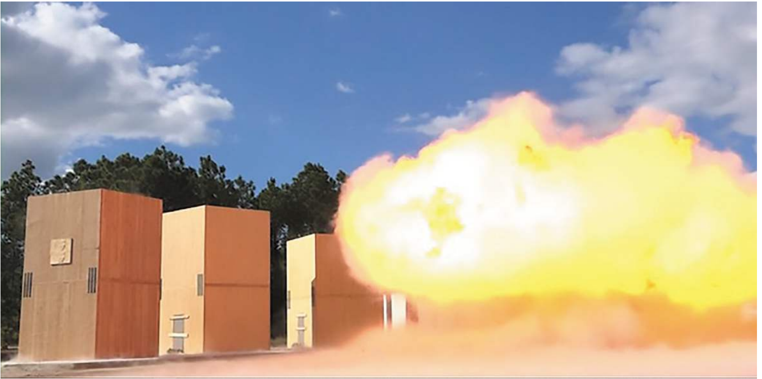
Blast Testing CLT. Use Photo from USDA press release: https://www.usda.gov/media/blog/2018/03/30/blast-testing-shows-clt-can-take-heat All three structures remained standing after the testing – even tests designed to take the structures well beyond their design intent. (Photo courtesy of Air Force Civil Engineering Center AFCEC, Tyndall Air Force Base)
