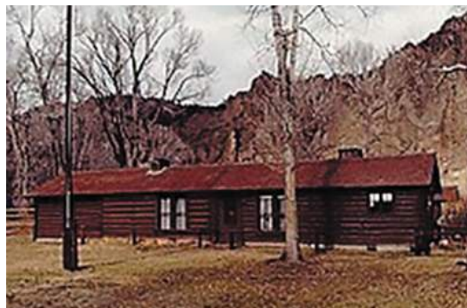
Wapiti Ranger Station
